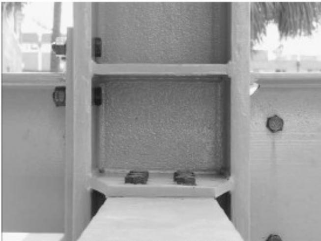
Figure 5-11. Moment Connection: Extended end-plate. Column C1 / Girder B3.
