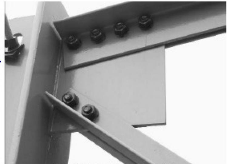
*Figure 7-17. Misc. Connection: Truss
