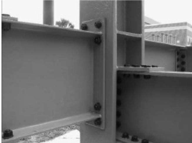
Figure 5-10. Moment Connection: Extended end-plate. Column C1 / Girder B3.
