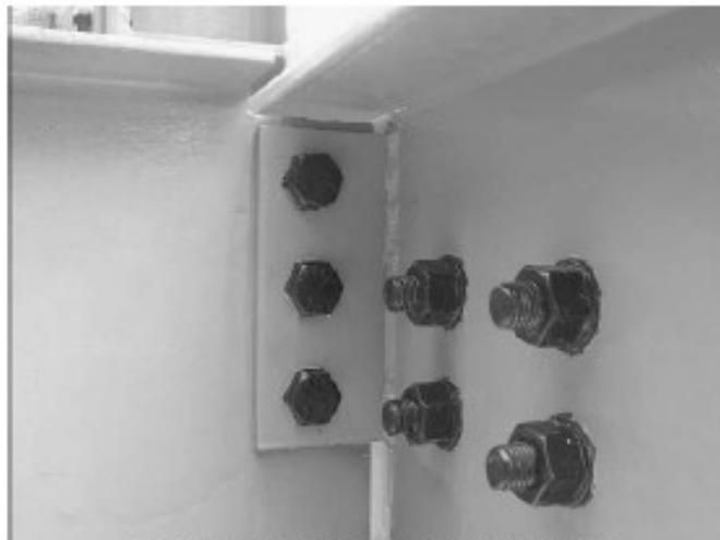
Figure 4-32. Shear Connection: Single plate
