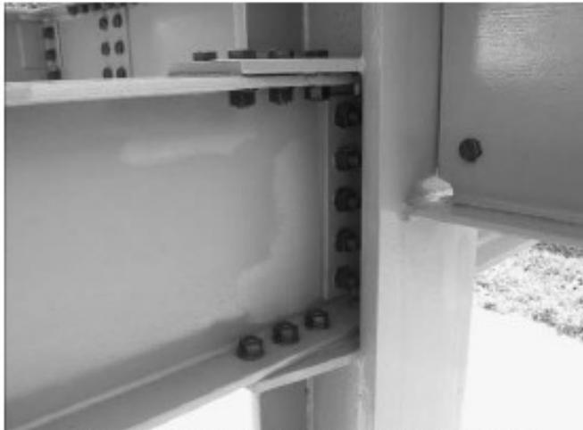
Figure 5-2. Moment Connection: Bolted flange plates
