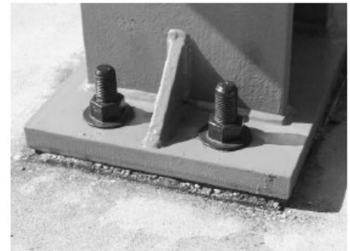
*Figure 6-7. Column Connection: Base plate
