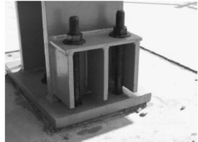
Figure 6-4. Column Connection: Base plate Foundation / Column C1
