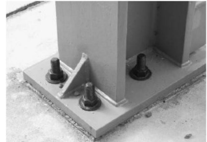
*Figure 6-6. Column Connection: Base Plate
