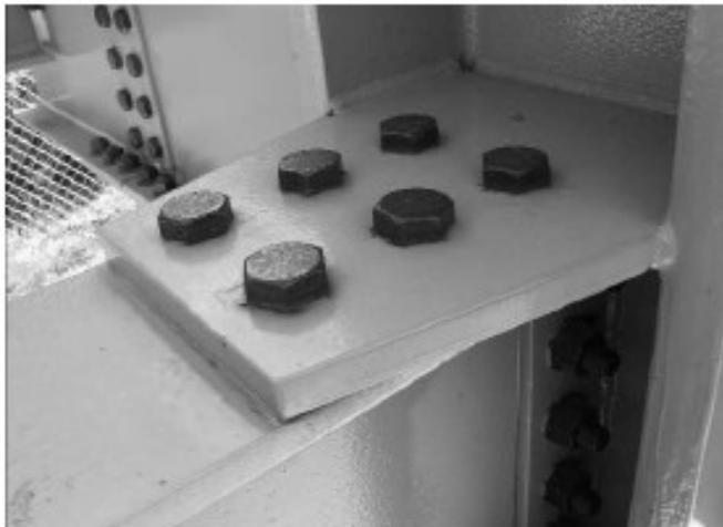
Figure 5-3. Moment Connection: Bolted flange plates
